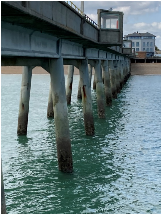
Supporting pier legs beneath pier stem and lower deck below.
