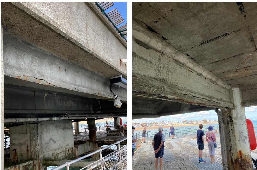
Supporting cross beams beneath Pier Café (lower deck).
